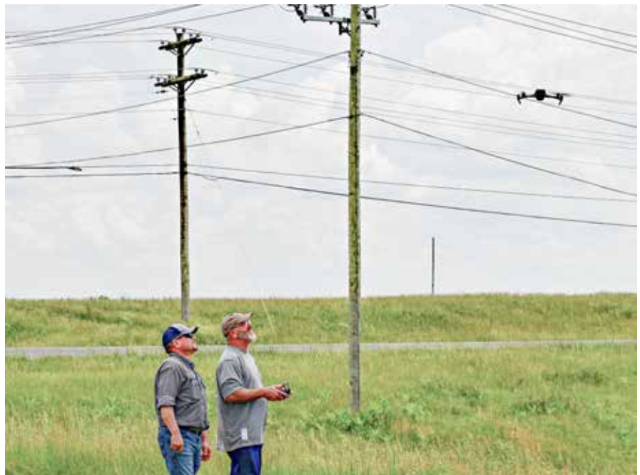
Service Technician Steve Moore and Line Inspector Travis Duvall survey power lines using Owen Electric's new drone technology. Photo: Whitney Duvall
