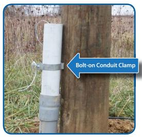
For services that involve an existing pole, a 3 ft. radius 90 degree elbow shall be used at the pole with conduit extending 2 ft. above ground and attached firmly to pole by a bolt-on clamp.
