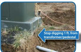
Conduit shall be 3 in. schedule 40 PVC (gray in color) and extend from the end of ditch to the meterbase. Anything above grade to meter base should be schedule 80 PVC per NEC 300.50(c). For services that come from a transformer/pedestal, stop conduit 1 ft. from transformer/pedestal. Conduit shall be covered at both openings to keep out water/debris, with end of ditch exposed.
