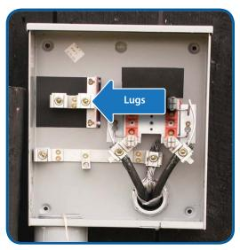
Meterbase shall be mounted at eye level (including finished grade). Conduit shall be mounted on same side of meterbase as lugs. Milbank brand meterbase preferred.
