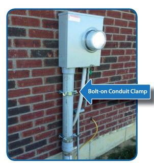
The conduit as well as an underground meterbase shall be firmly fastened to structure. Conduit shall be fastened by a bolt-on clamp with at least a 2 in. lag screw. A pull string shall be installed throughout the entire length of the conduit.
