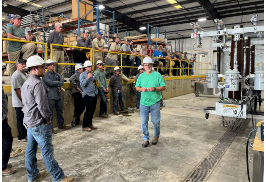
Charlie Lewis and Kevin McCarty with Kentucky Electric Cooperatives conduct transformer bank training with Owen Electric construction crews. Photo: Trevor Evans
